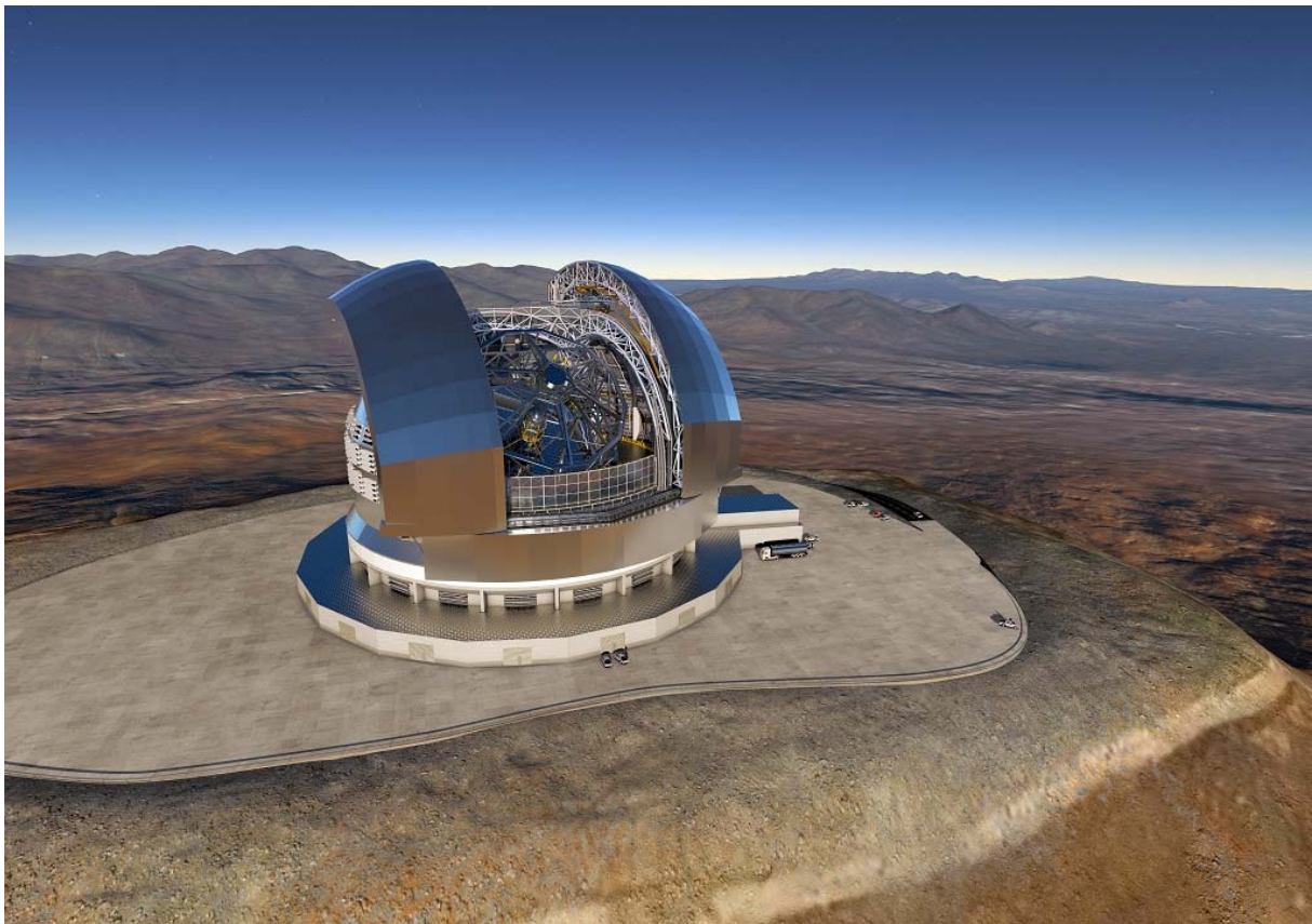
Fig.1: Flagship of European astronomy, the 39-meter Extremely Large Telescope under construction.
